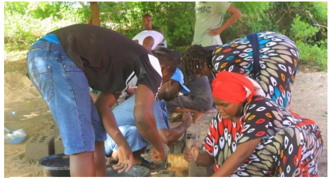
Community members engage in the construction of restorative materials to aid in these efforts.
